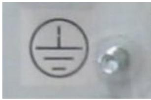
Fig. 23: Grounding stud marked with PE symbol
